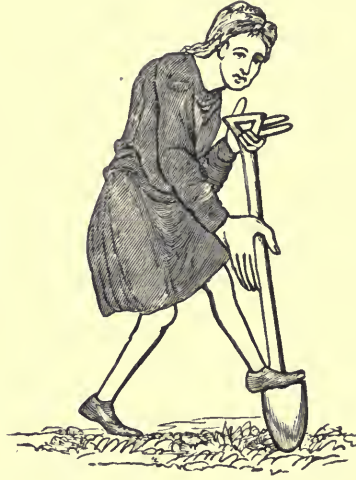
DIGGING. Eleventh Century. MS. Cott. Claud. B. iv.
